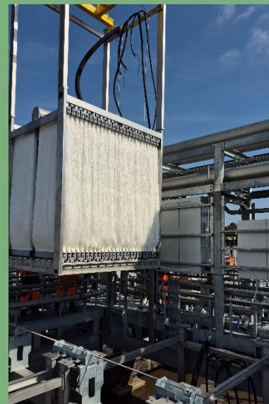
Figure 1 – ZeeLung cassette during installation in anoxic tank
